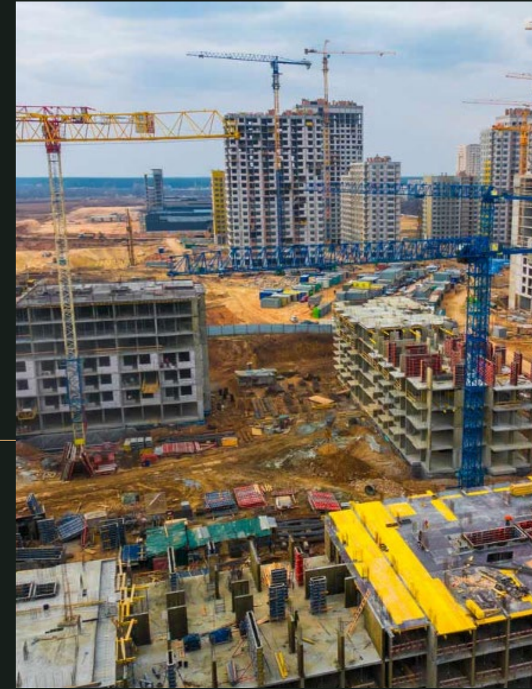
CONSTRUCTION & SITE CONTROL
